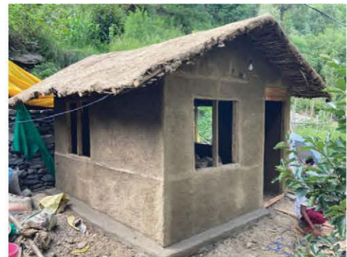
Wattle & daub hemp hut
